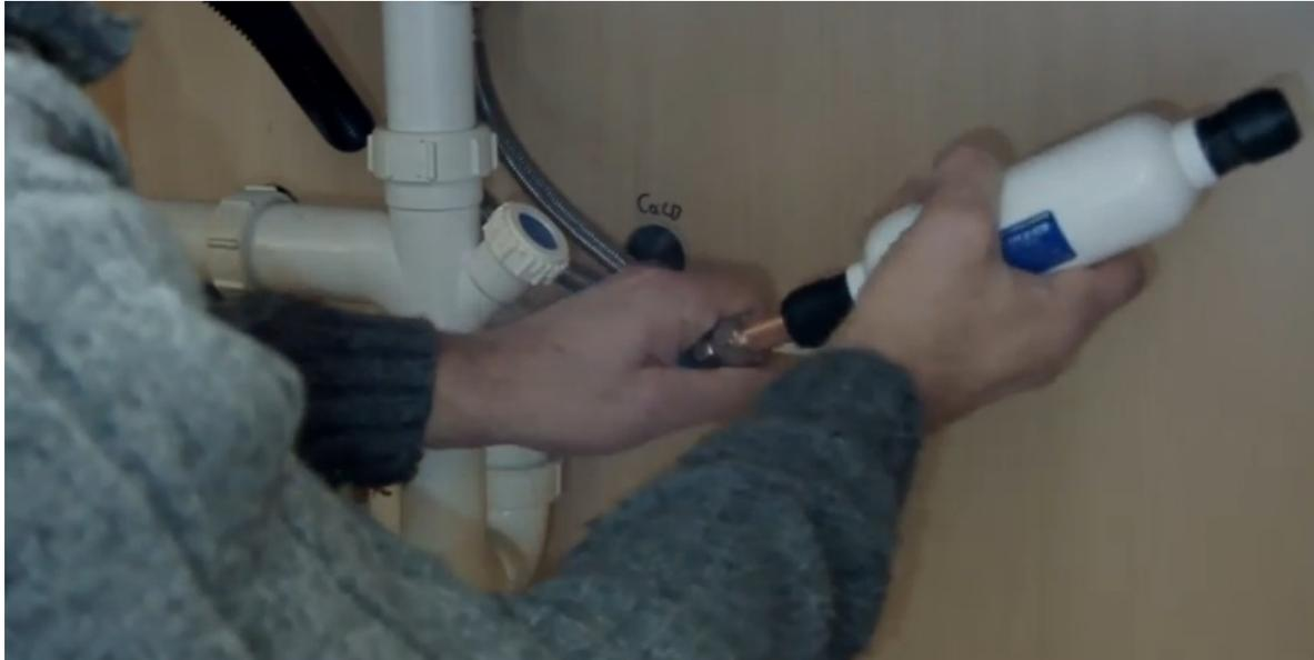
The filter has a flow arrow pointing in the direction of the water flow. This indicated where the “in” and “out” goes, so ensure you have the filter pointing in the right direction for your water flow. Your filter comes with a mounting clip which you can position accordingly.
