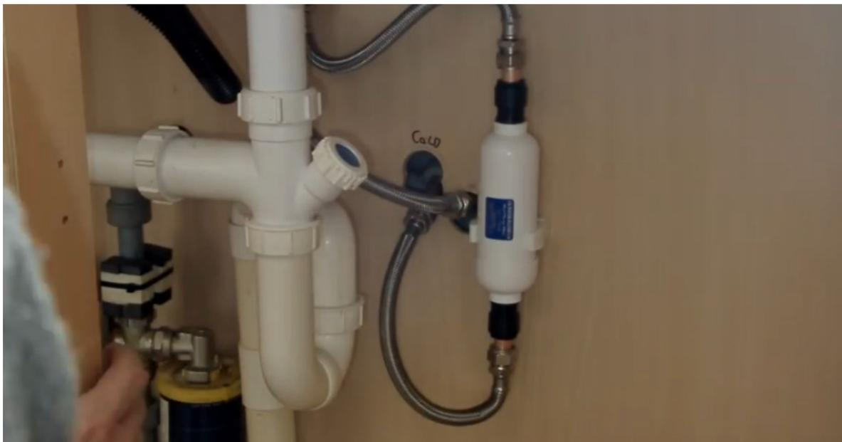
Once the filter is in position, you can turn on the cold water supply and check for any leaks. Run the filter for at least 5 minutes to flush the filter of any loose carbon or sediments.
